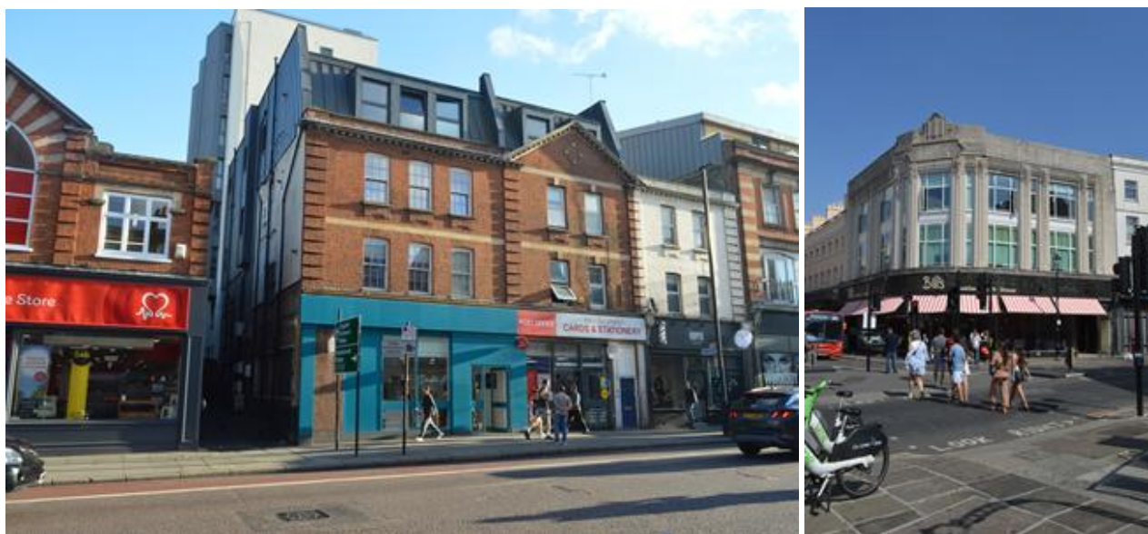
3. 1918. 157 High Street, Wandsworth, SW18. The corner shop which was Burton’s first in London. Clearly pre-existing. Any Burton embellishment must have been restricted to the shop front.
