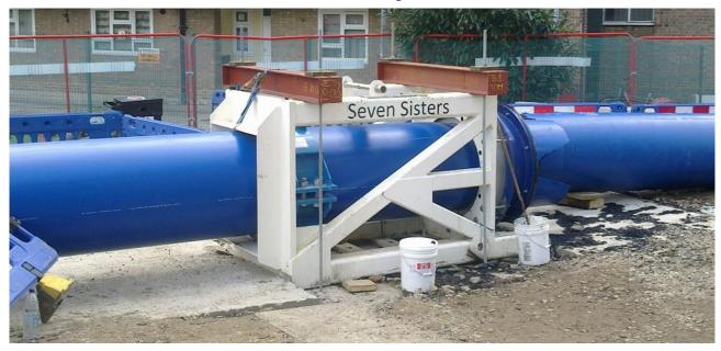
This slightly reduced the diameter of the lining when held in tension. Two men added lubricant from a pair of white cans (see photograph above) while this was taking place. The process was one of drawing, like wire, rather than extrusion like toothpaste. The linear winch consisted of two hydraulic rams pulling in alternation. Their safe working capacity was 100 tonnes force but in practice the tension was about 49 tonnes.
