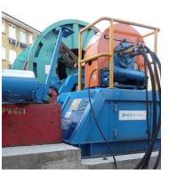
From the end of the section of main being lined, a powerful linear hydraulic winch (above centre) hauled the lining through the main by a heavy wire rope, aided by a rotary hydraulic winch driving a drum to take up the slack in the rope (above right). As the plastic lining entered the main it was first drawn through a metal die mounted in a substantial welded steel frame anchored to the ground, see below.
