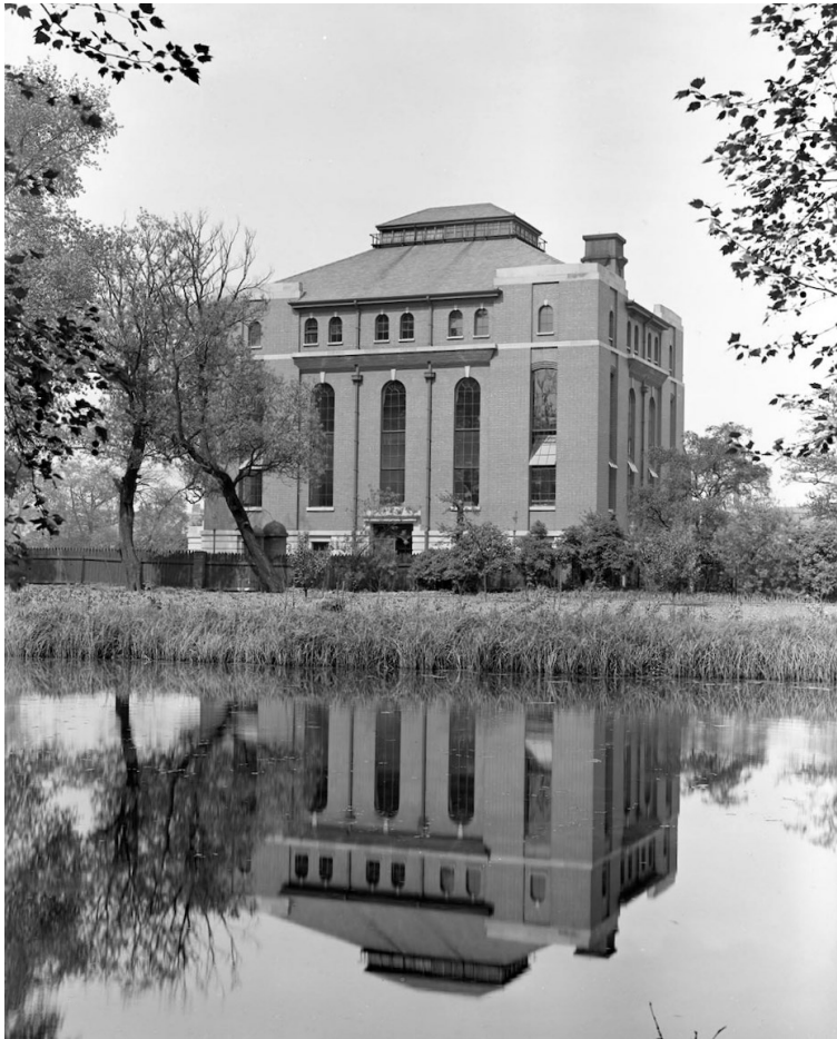
Left above: James engine house at Brookmill, now in Beck Close, SE13 and still operational
