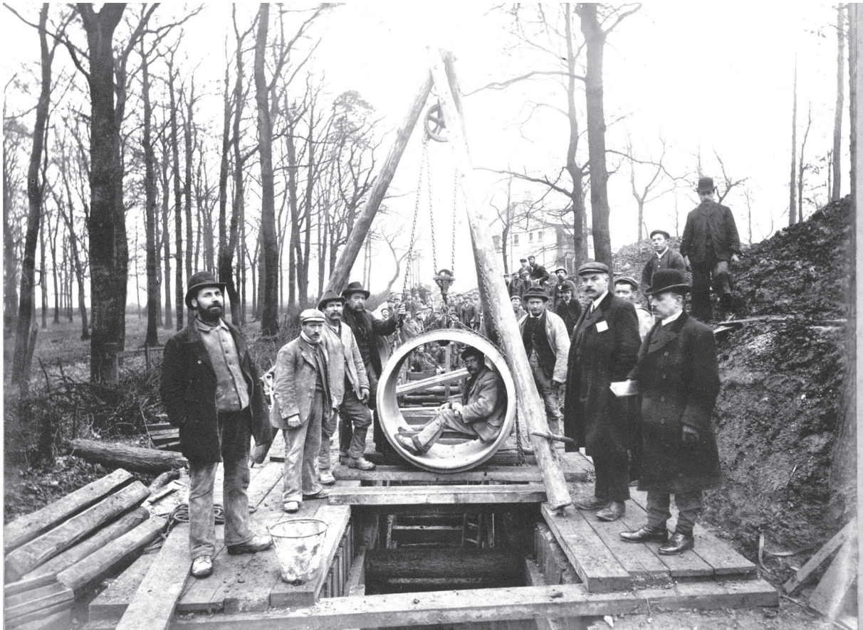
Figure 1. Workmen laying a sewer pipe at an unknown location in Finchley in the late nineteenth century. Courtesy of Barnet Local Studies
